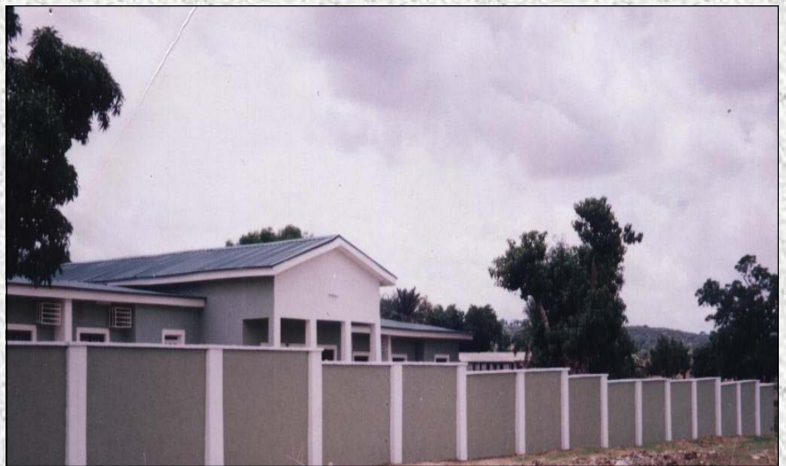
Pictures above: A section of TRCN zonal offices under construction.
